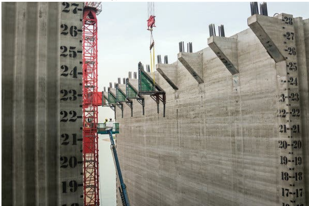
Caissons, or watertight retaining structures, that are part of the project.Credit...Sim Chi Yin/VII, for The New York Times
